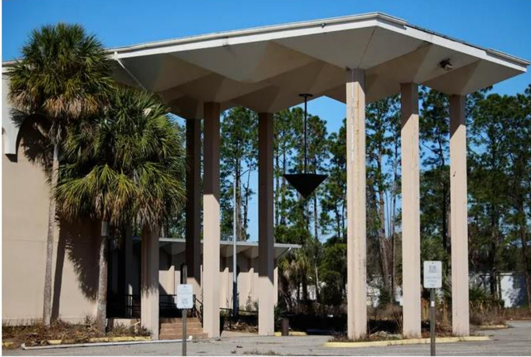
The Morocco Shrine Center was demolished in February to make way for the Village of Town Center mixed-use project. The development will span 37 acres and be home to over 1,000 residential units along with retail, restaurant and office space. Corey Perrine/Florida Times-Union
